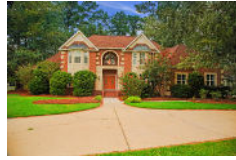
4207 Sweet Gum Crossing North Charleston SC
